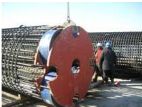
Multiple O-cell Assembly ready for installation
