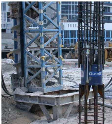
Test pile being constructed and O-cell assembly ready for installation
