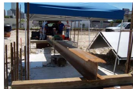
Test in progress under the reference beam
