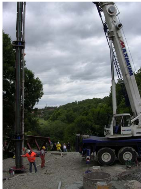
Lifting of the steel frame showing two O-cells at two levels
