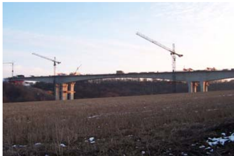
Bridge construction progress March 2006
