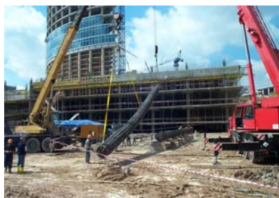
Reinforcing cage with O-cell installed
