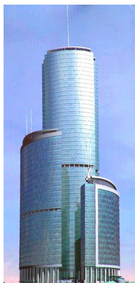
Naberezhnaya Tower C
