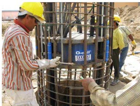
Installation of one of the O-cell assemblies
