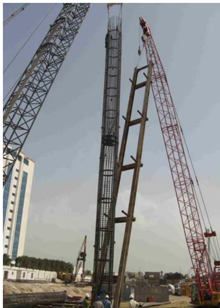
Lifting of O-cell assembly prior to installation
